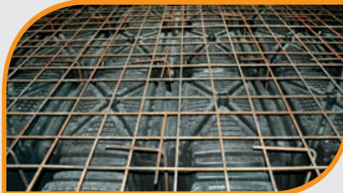
In heights 60-65-70 cm, GRANCHIO is equipped with fixing keys that ensure improved grip for the legs during the casting of the concrete.
